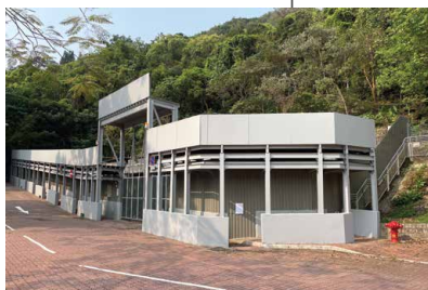
完成拆卸工程 Demolition Works Completed
